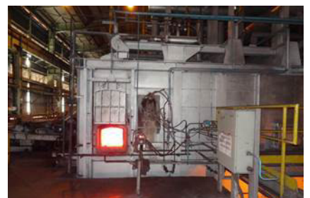
FurnaceSpection system setup
