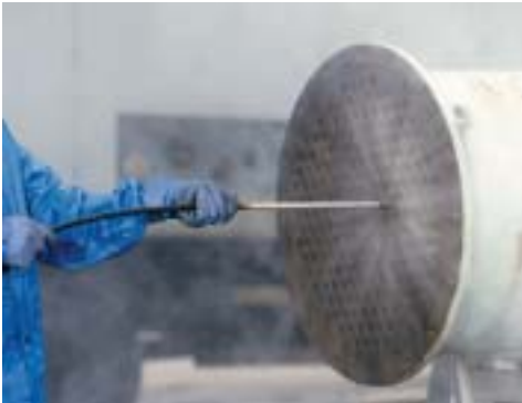
Cleaning of heat exchanger with Spin Nozzle.
