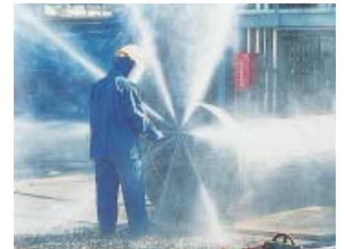
Cleaning of heat exchanger with Lance Nozzle.
