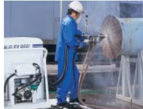
Inner surface cleaning of heat exchanger tubes by Flex Reel.
