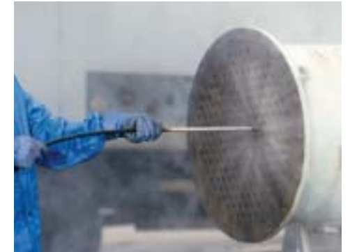
Cleaning of heat exchanger with Spin Nozzle.
