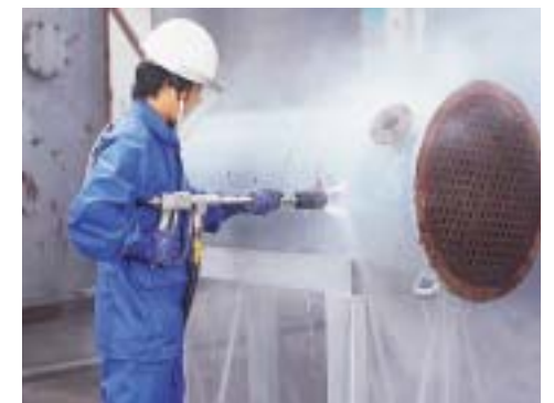
Outer surface cleaning of heat exchanger by Grip Jet Gun with V-Rotary Nozzle.
