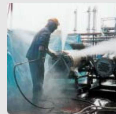
熱交換器の内面洗浄 Cleaning of Heat Exchanger Tube Inside
