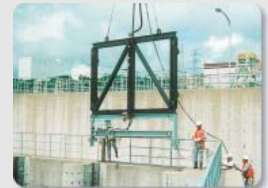
取水口戸当り部洗浄 Cleaning of Water Intake Gate
