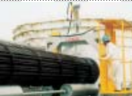
熱交換器の外表面洗浄 Cleaning Outside of Heat Exchanger Tubes
