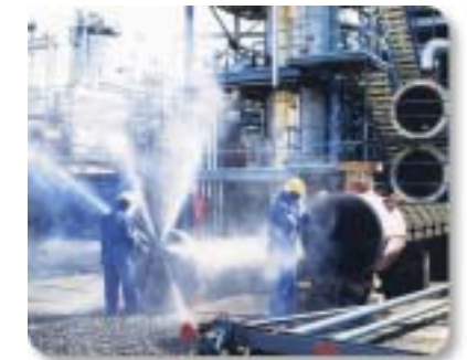
熱交換器のチューブ内面洗浄 Cleaning Inside of Heat Exchanger Tubes
