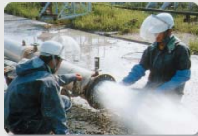
大口径管の洗浄 Cleaning of a Large Pipe
