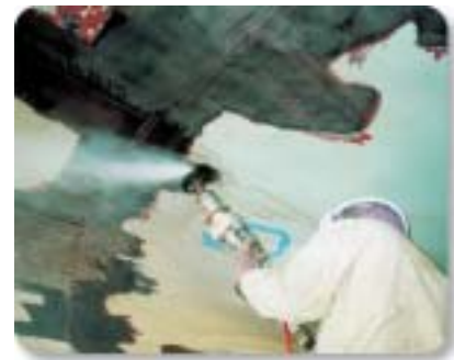
球形タンクの塗膜はくり Removal of Paint from Spherical Gas Tank
