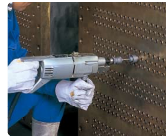
Tube expansion with tube rollers
