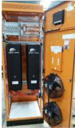
AHF rated 415V 50Hz -288kvar to +288kvar
